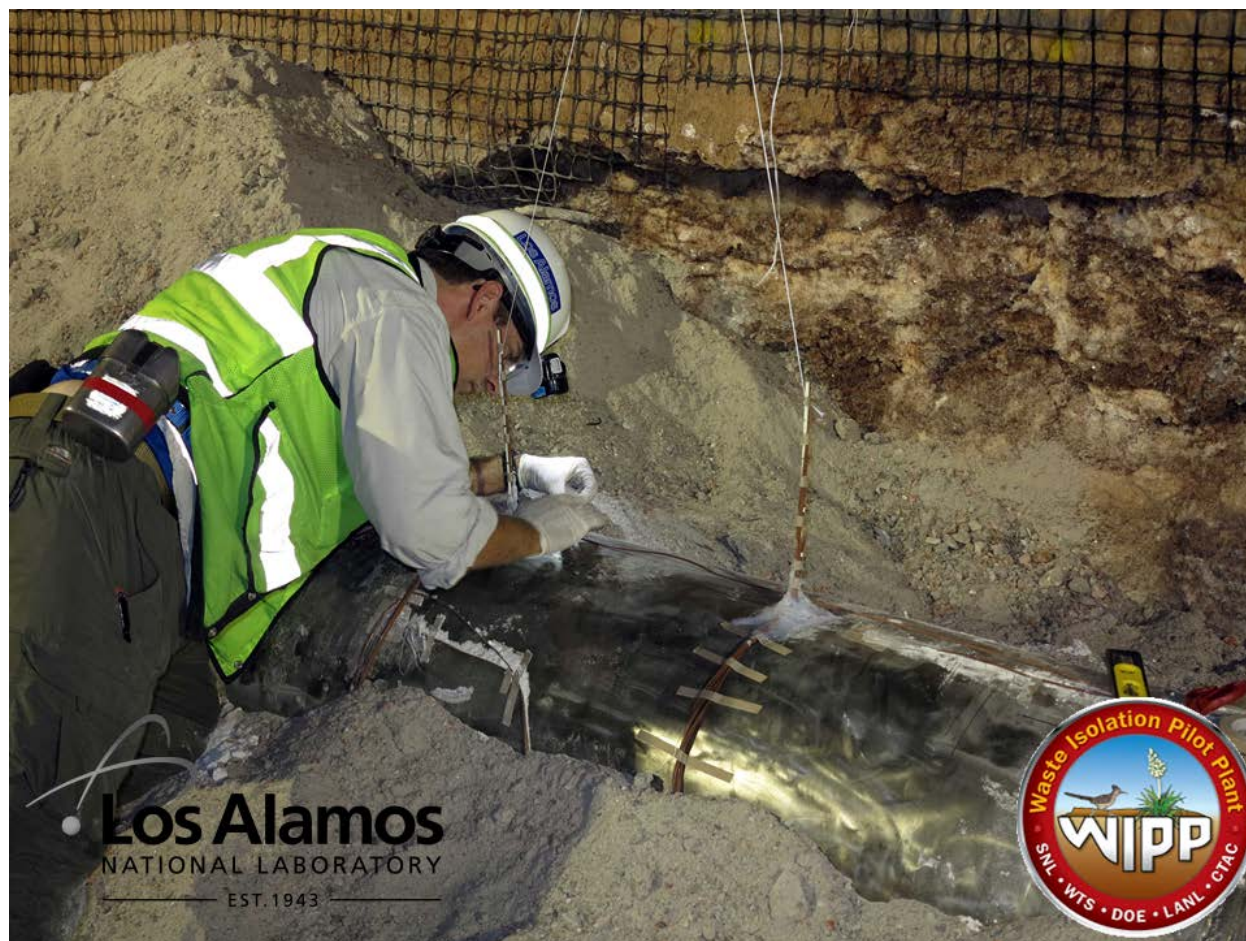
Figure 51: Installation of vertical thermocouple arrays extending from top of can towards top of pile.
