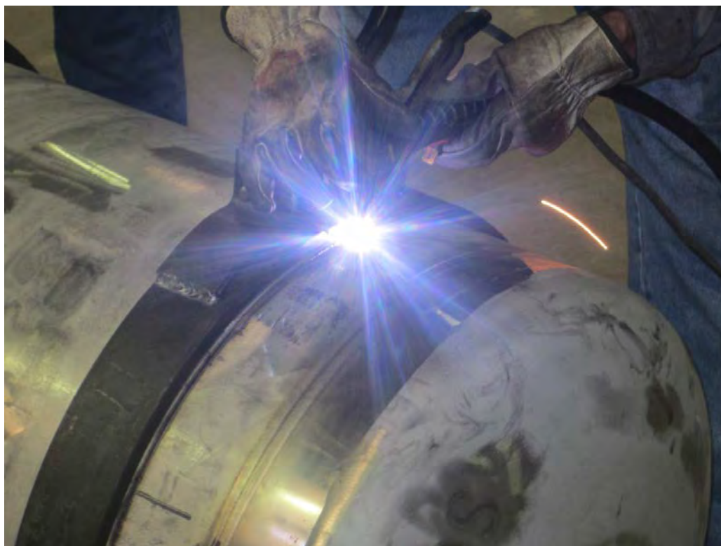
Close Up of Cut in Progress
