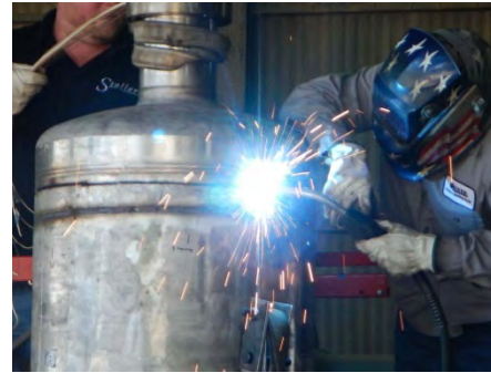
Figure 6: Reattaching pintle end
